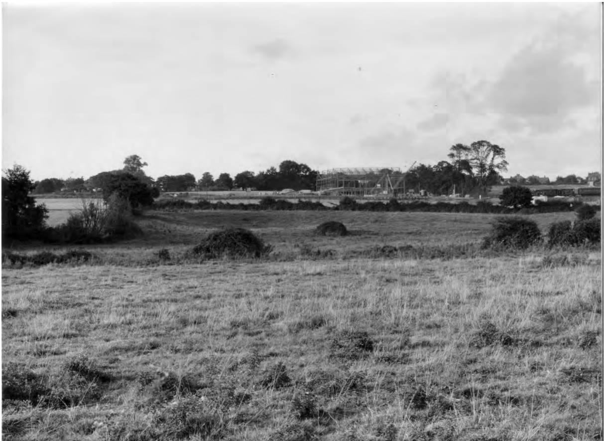
A new building going up. September 1937.
